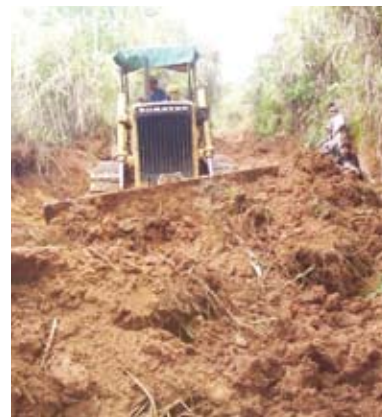
Road works, Pao, Philippines
