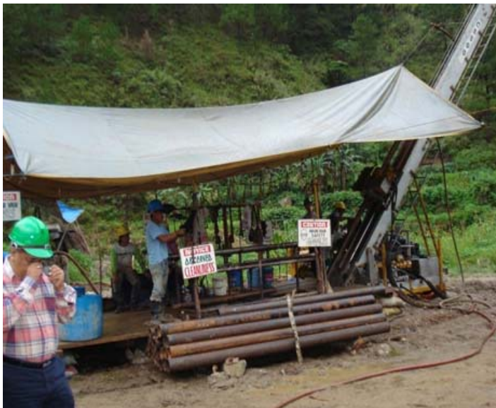
First drill hole at Gambang
