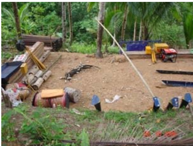
Site of the first drill pad at Malangza.
