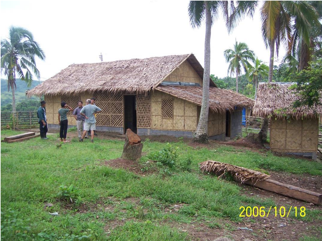
Newly constructed Drillers camp and facilities at Samay
